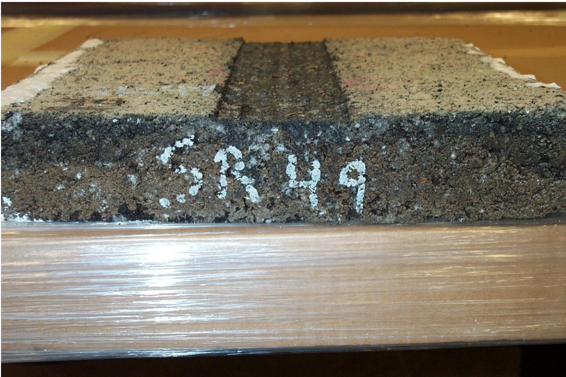
Figure C2 SR 49 after Purwheel Testing
